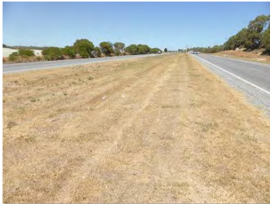
Figure 8: The mown grass fuels in the middle of the dual carriage way – Mandurah Road.
